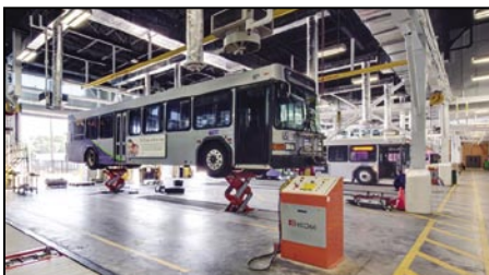
^ GRTC BUS MAINTENANCE FACILITY, RICHMOND, VA
